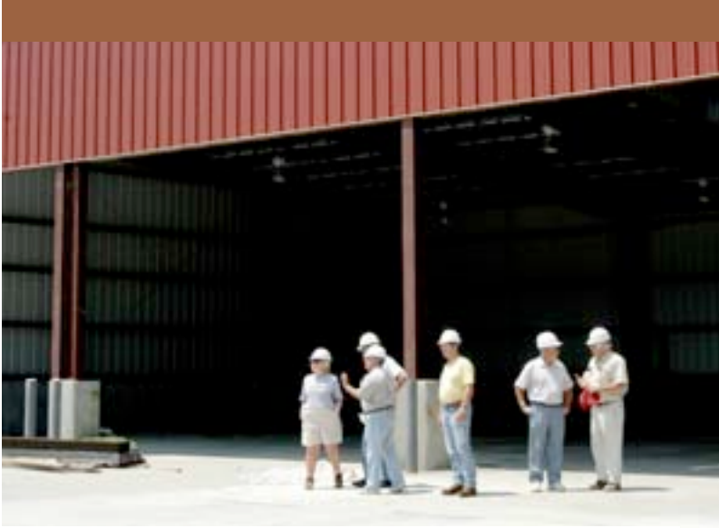
DSWA staff and Board tour improvements to the Pine Tree Corners Transfer Station
