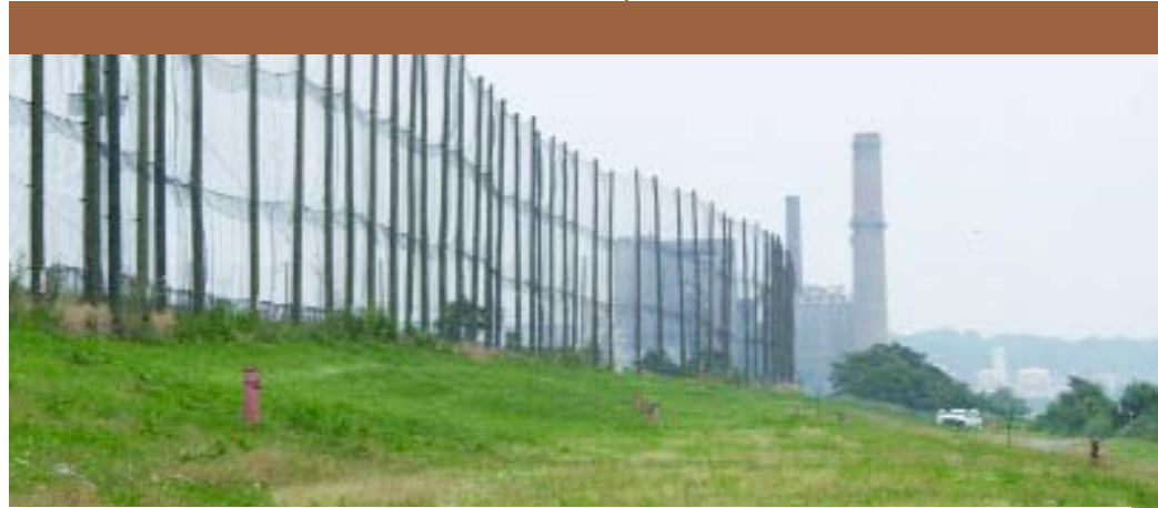
Environmental protection at the Cherry Island Landfill includes the use of this litter fence designed to keep windblown debris from leaving the site.
